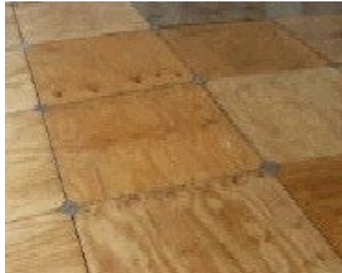
Laydown Plywood Flooring
